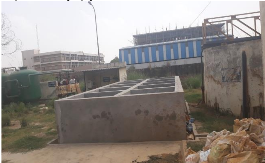
Newly Constructed Sludge Drying Beds & Concrete Pads
