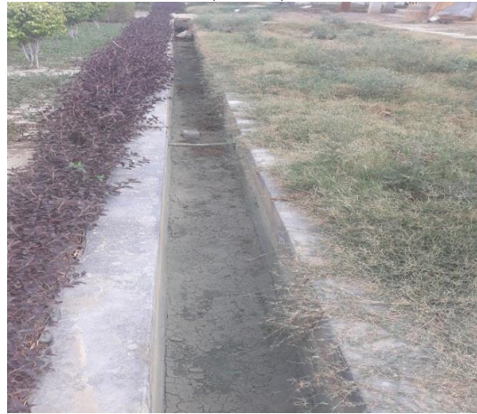
Storm Water Drains ( After )
