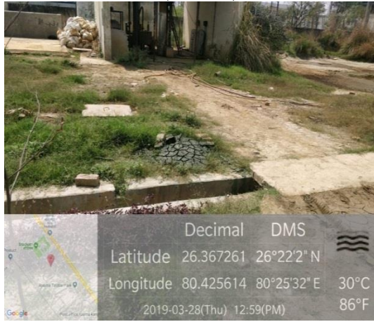
Storm Water Drains ( Before )
